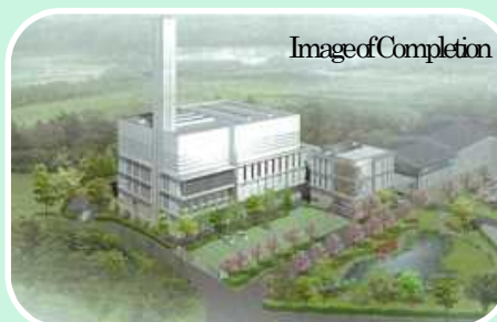
Sukagawa area New garbage disposal site
